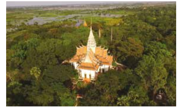
10 Wat Traleang Kaeng, at Longvek, Kompong Chhnang province.
