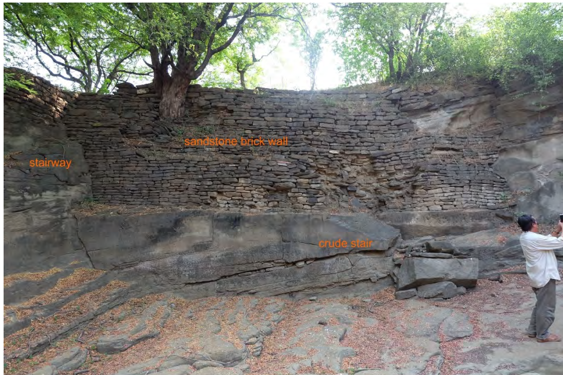
Fig 9. Northeastern stairway, symbolic stairway (crude stair), and sandstone “brick” wall enclosing the eastern side of Nat Yekan tank (note quarry scars in the lower left corner of the photo). Source: Gyles Iannone
