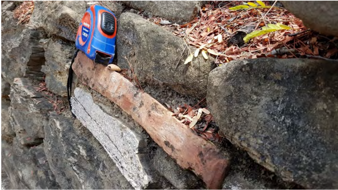
Fig 15. Early Bagan Period brick in the east wall of Nat Yekan tank. Source: Gyles Iannone
