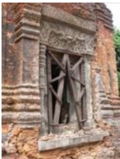
Photograph 6.51 Doorway of Prasat Lolei supported with props
