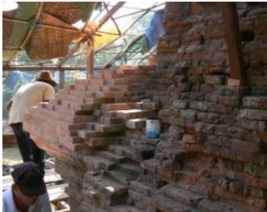
Photograph 6.53 Preah Ko tower showing the original section before restoration (2006)
