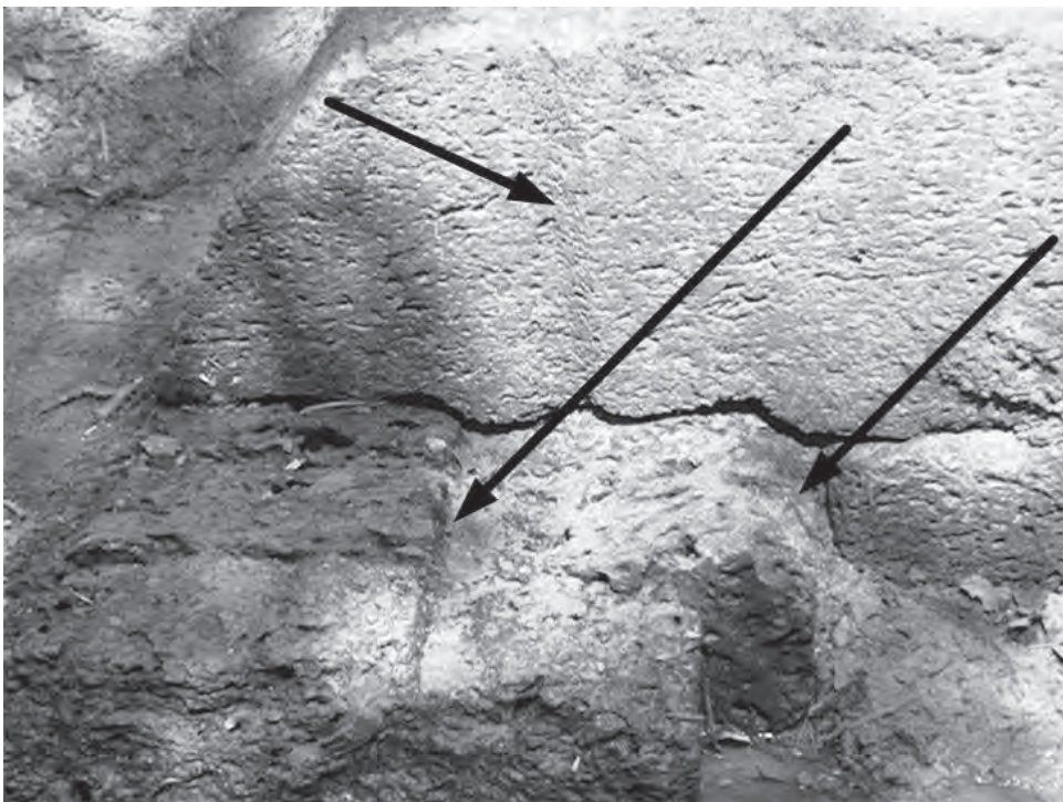
Figure 7 Vertical and horizontal keys in spillway construction.
