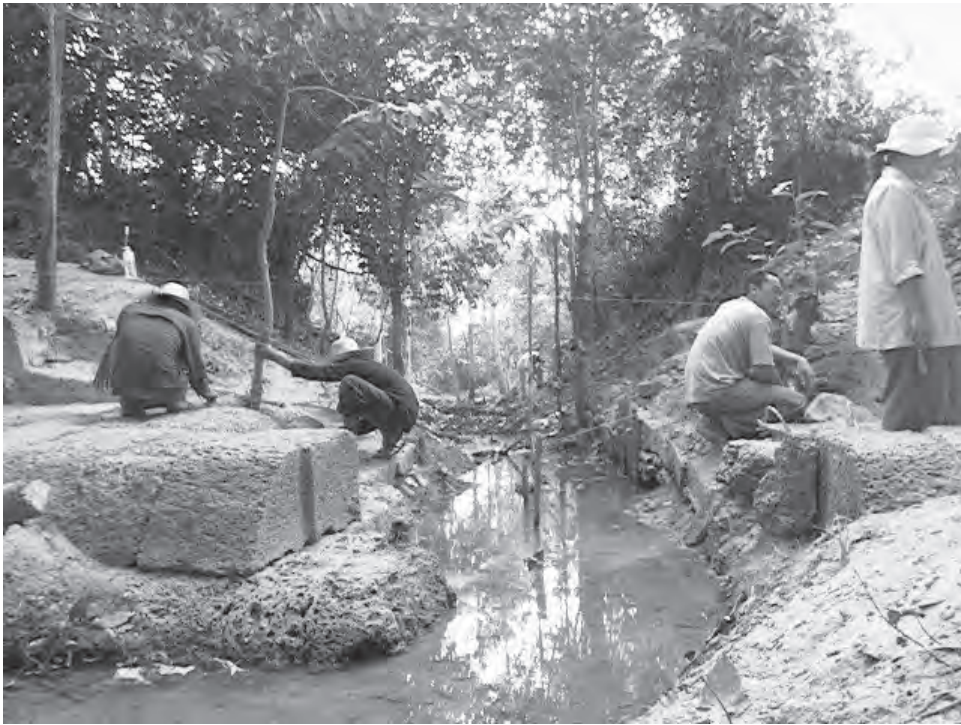
Figure 6 Spillway and Bam Penh Reach channel. Excavation nearby indicates base of spillway is about 1½ m below the crest.
