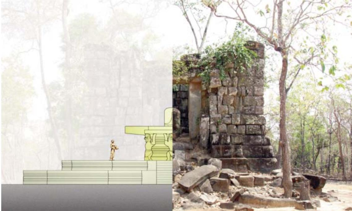
*Figure 4: Conjectural initial phase of the monument KK8 before constructing the wall on its platform (left half), and present condition (right half). Three shrines KK7 (Prasat Balang), KK8 (Prasat Thneng), and KK11 (Prasat G) that are aligned on a perpendicular line of the main axis of Prasat Thom, are quite similar in architectural design and show signs of unfinished renovation.*
